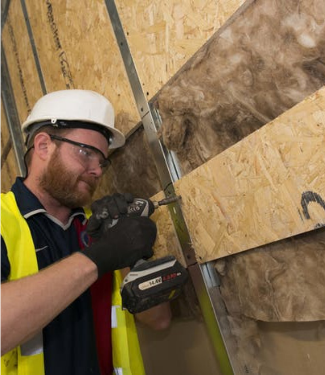
Installation of pattressing
