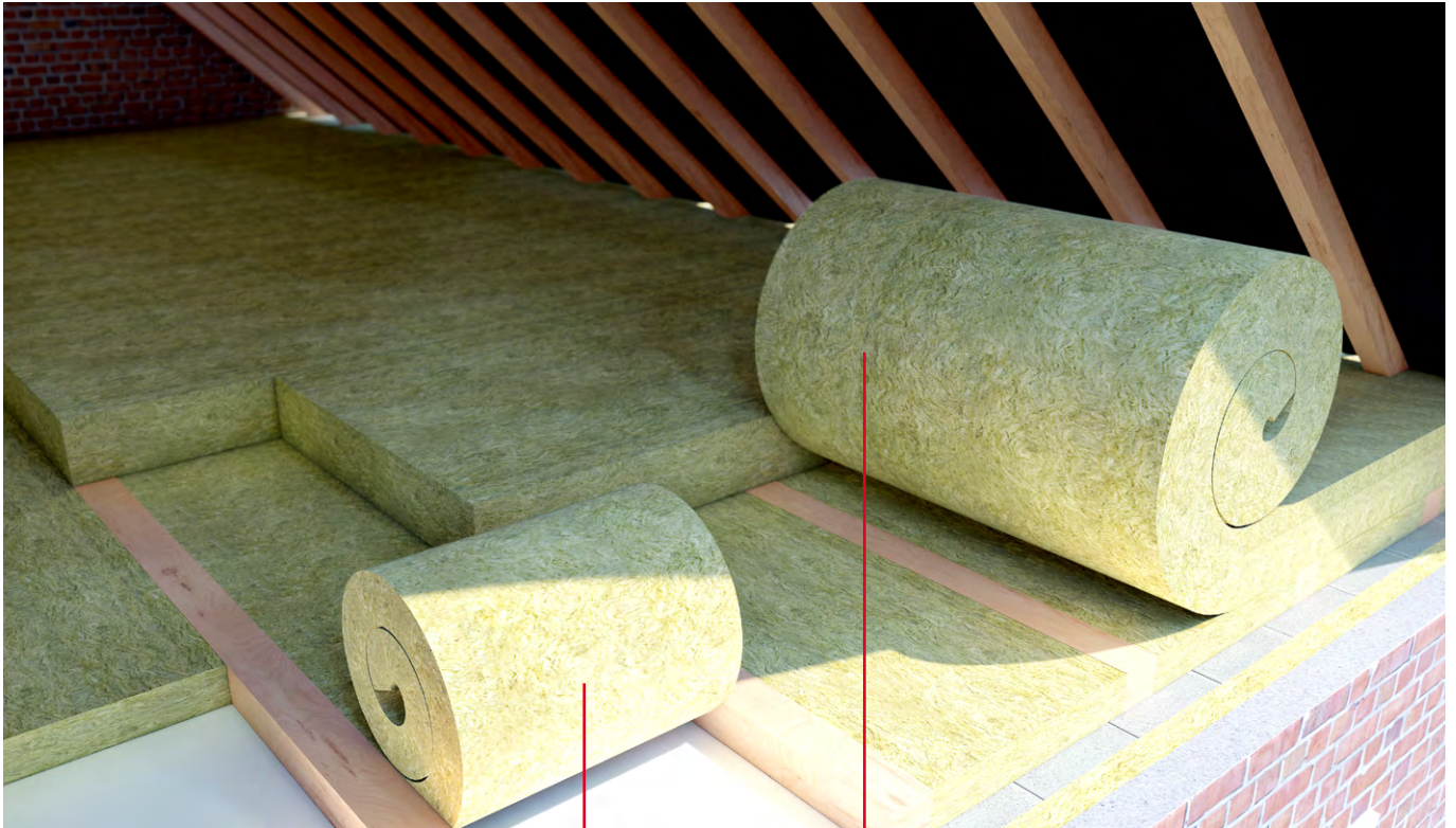
Thermal Insulation Roll laid at 100mm thickness in between the joists
